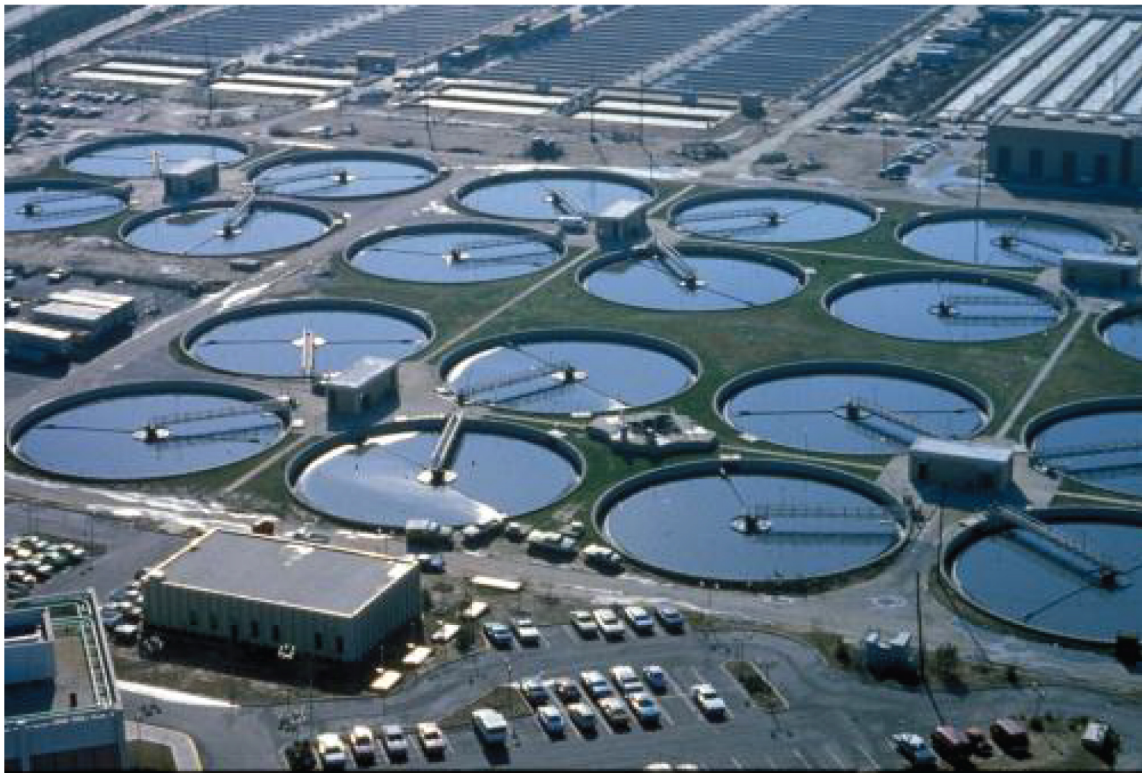
Sewage Treatment Plant
