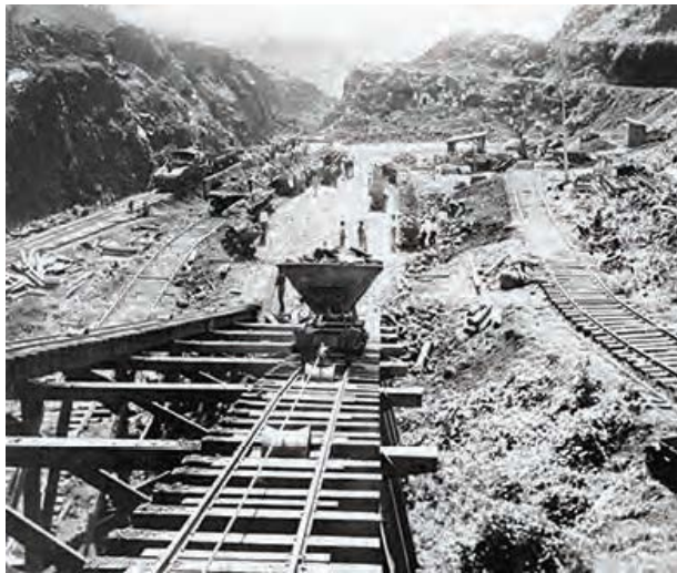
Figure 35 Recurring landslides made the excavation of the Culebra Cut one of the most technically challenging elements in the construction of the Panama Canal.
